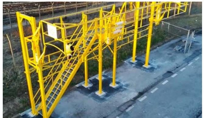
3.2a Inspection gantry for top access to tank
